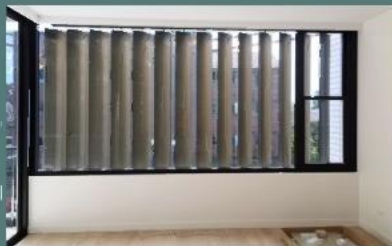
Product: Aluminum shading louver - oval Material: Aluminum alloy Photograph: Australian completion project site Open: Manually open + fixed Applicable: office/hospital/shopping mall aisle, laundry room, rest area
