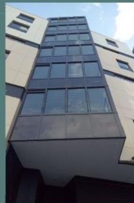
Products: Glass shutter Material: Aluminum alloy + single glass Photograph: Australian completion project site Enable: Manually enable Applicable: office/hospital aisles, shopping malls, laundry rooms
