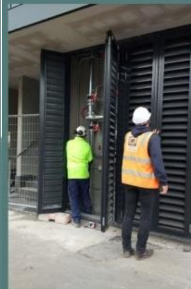
Products: Aluminum alloy louver bevel Material: Aluminum alloy Photograph: Australian completion project site Open: Fixed + manual door and window louvers
